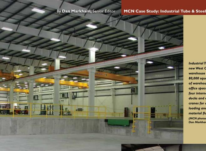
Industrial Tube & Steel's new West Chester warehouse features 80,000 square feet of warehouse and office space with four internal loading docks and overhead cranes for quick loading and improved material flow. (MCN photos by Dan Markham)
